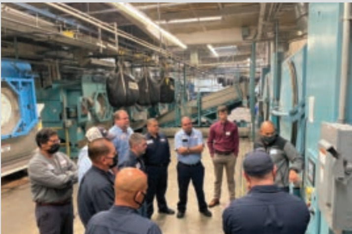
Dryer Controller Training
