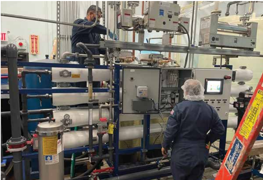
New skid mounted Reverse Osmosis upgrade installed in Richmond, VA plant.
