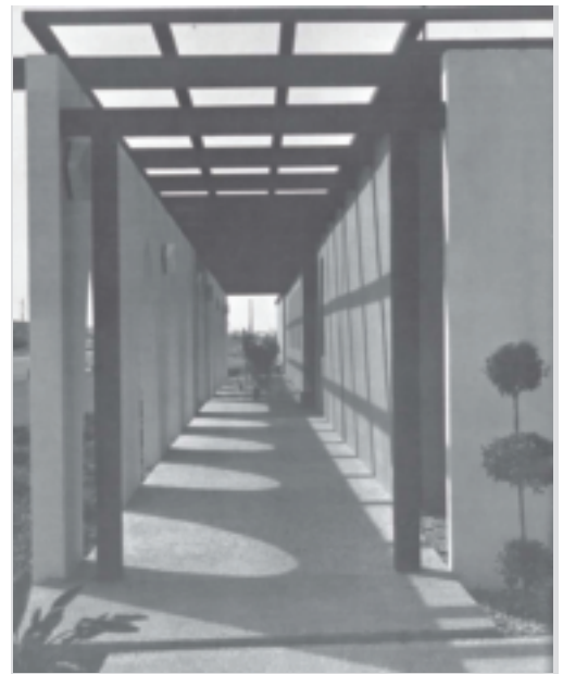
Original entry walkway.
