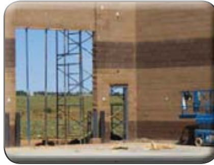
Inside of northwest wall
