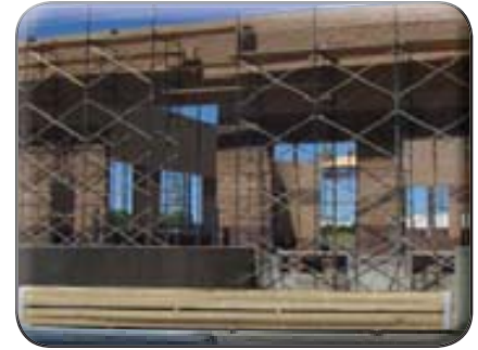
Roof deck material
