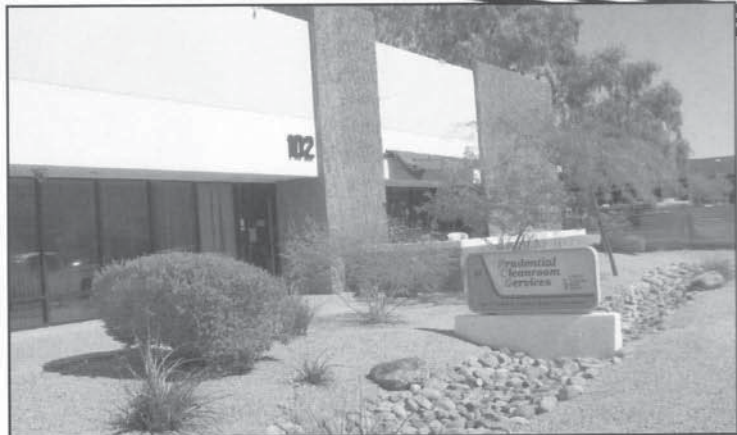
Mesa Cleanroom Plant 2006
