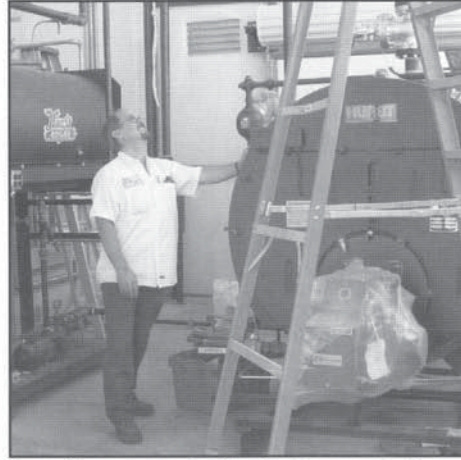
Installing a new boiler in the new boiler room addition.
