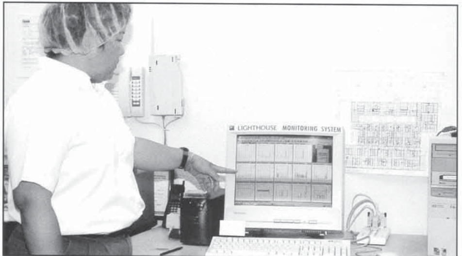
Kathy Araki demonstrates the Environment Monitoring system in place at Milpitas. The systems monitors levels of heat, air, water and other environmental factors.
