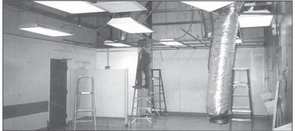
The old Distribution Area being torn down.
