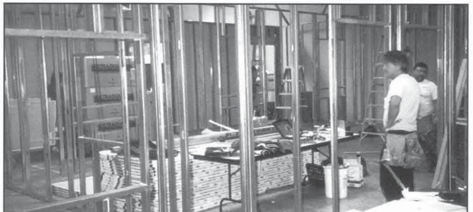
Temporary Cleanroom construction underway.
