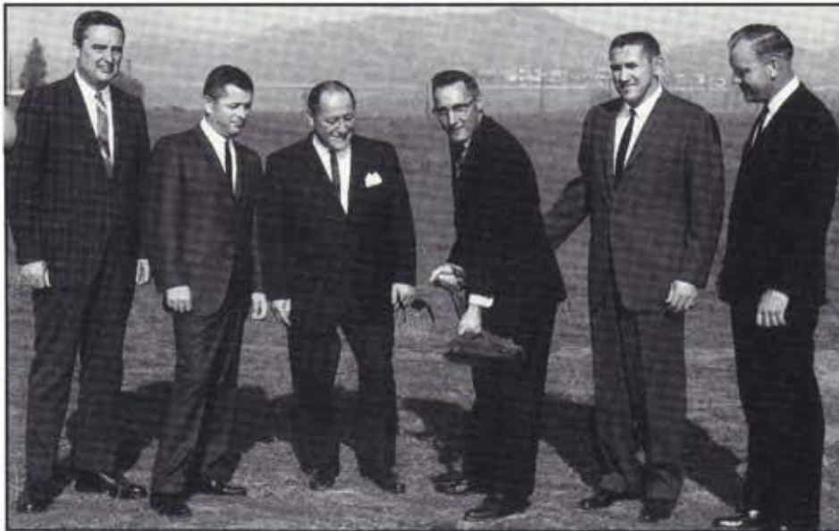
Ground breaking ceremonies for the original Riverside plant were held December 9, 1965. Holding the shovel is Clive Ruka, the first General Manager of Riverside. Don Clark is to his right.
