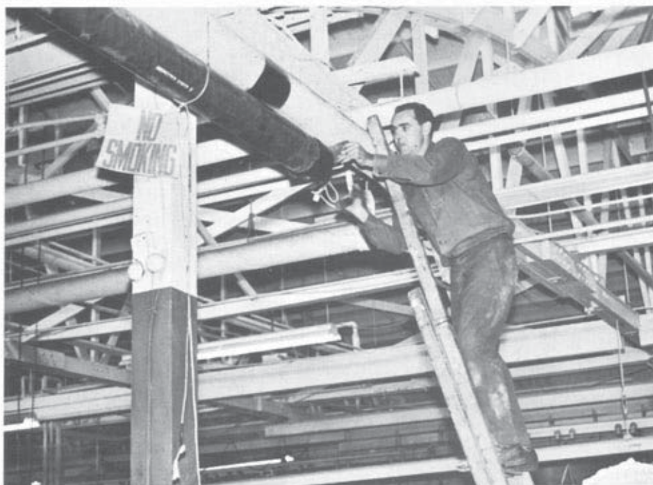
NEW WATER MAIN - Blair Gallagher, Company Engineer, pounds a section of pipe into place to complete a new 6" overhead water main in the Los Angeles Plant.
