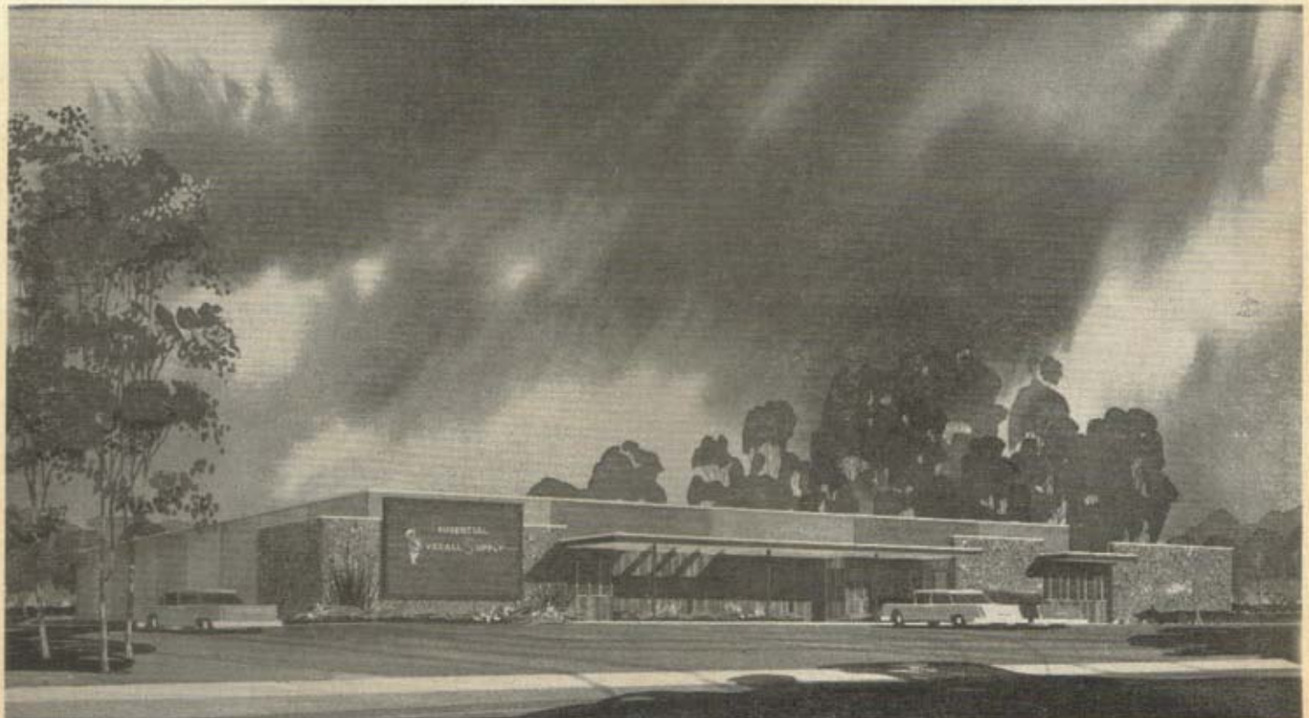
Artist's Conception of a New Industrial Laundry Now Under Construction by Prudential Overall Supply in the City of Riverside, California.
