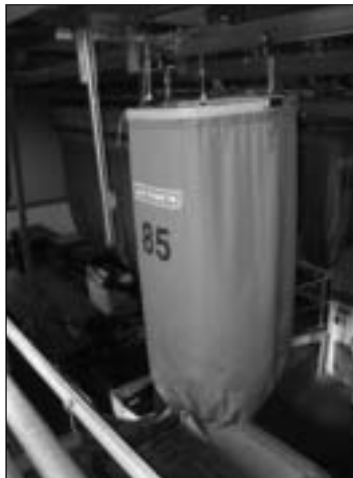
Overhead Rail Systems – Slings travel along rail systems automatically to load washers.
